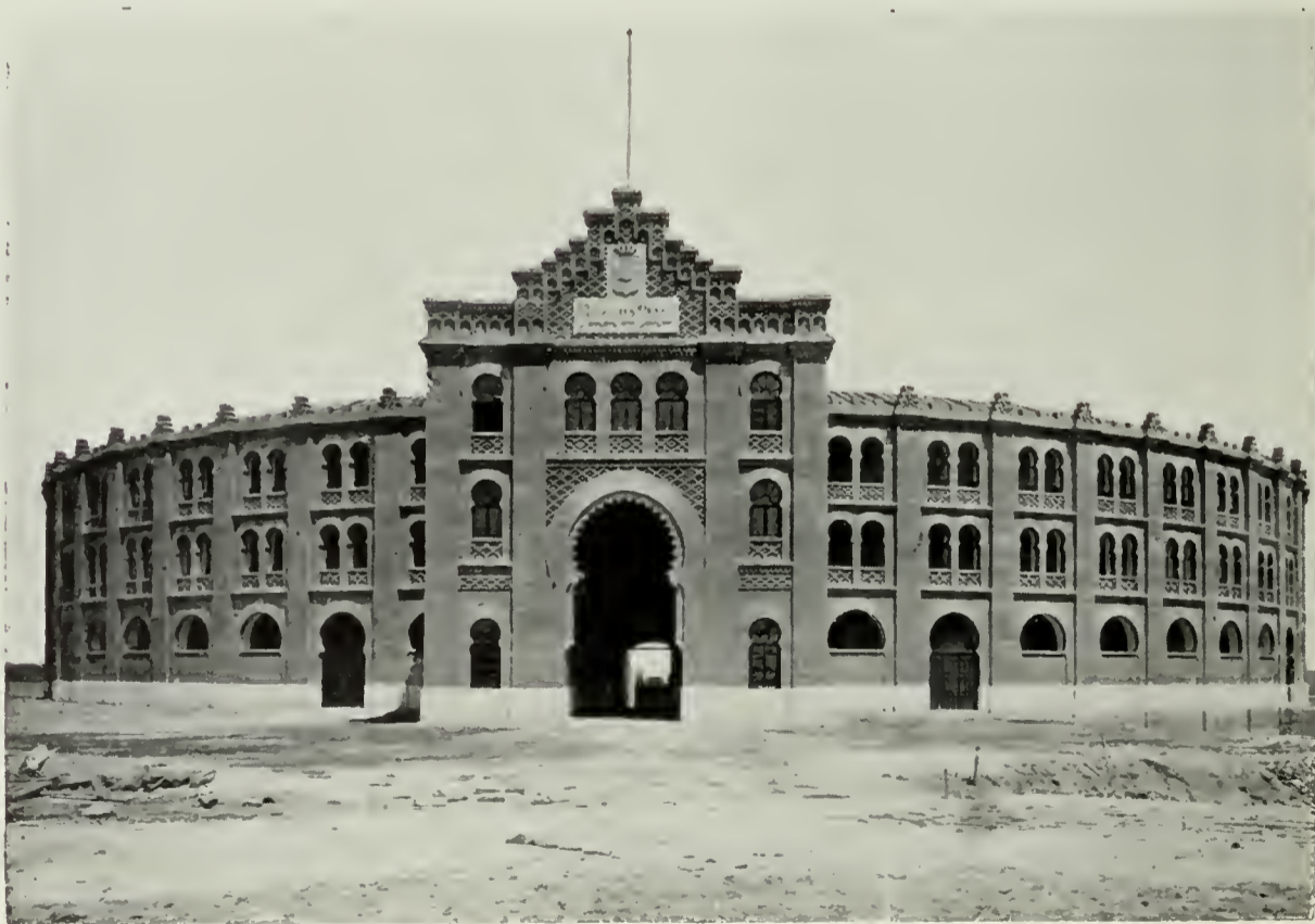
PRINCIPAL FAÇADE OF THE NEW "PLAZA DE TOROS," MADRID
